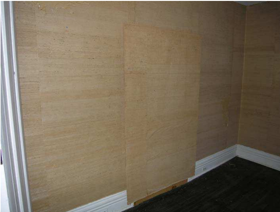
Master bedroom/dining room wall, showing the closed doorway.
