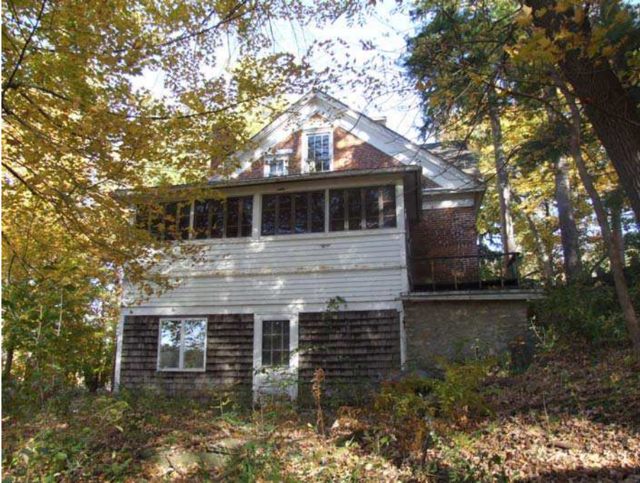
Figure 4. View from near the spring house (see lower level floorplan for photo vantage point). The sunroom was part of a 1930s remodeling and the cellar was built at an unknown date.
