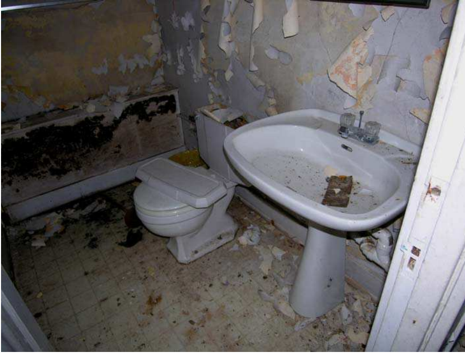
Figure 6. Lower level bathroom (see lower level floor plan for photo vantage point).
