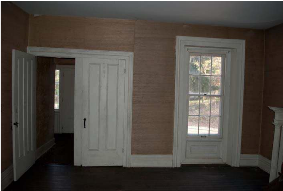
Figure 11. Main floor living room, looking into the front vestibule. The door to the right of the room's entrance leads to a closet (see main level floor plan for photo vantage point).
