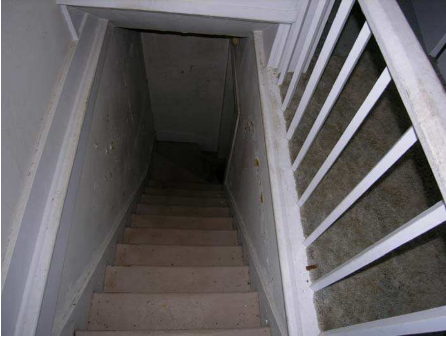
Stairway from the main floor to the upper level
