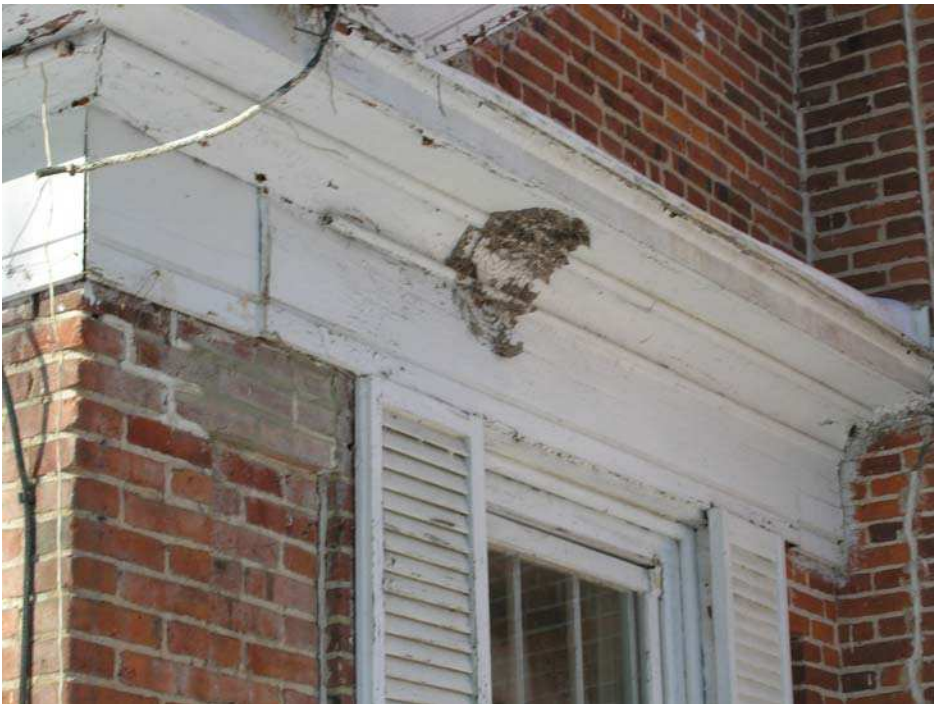
Southeast view of corner detail.
