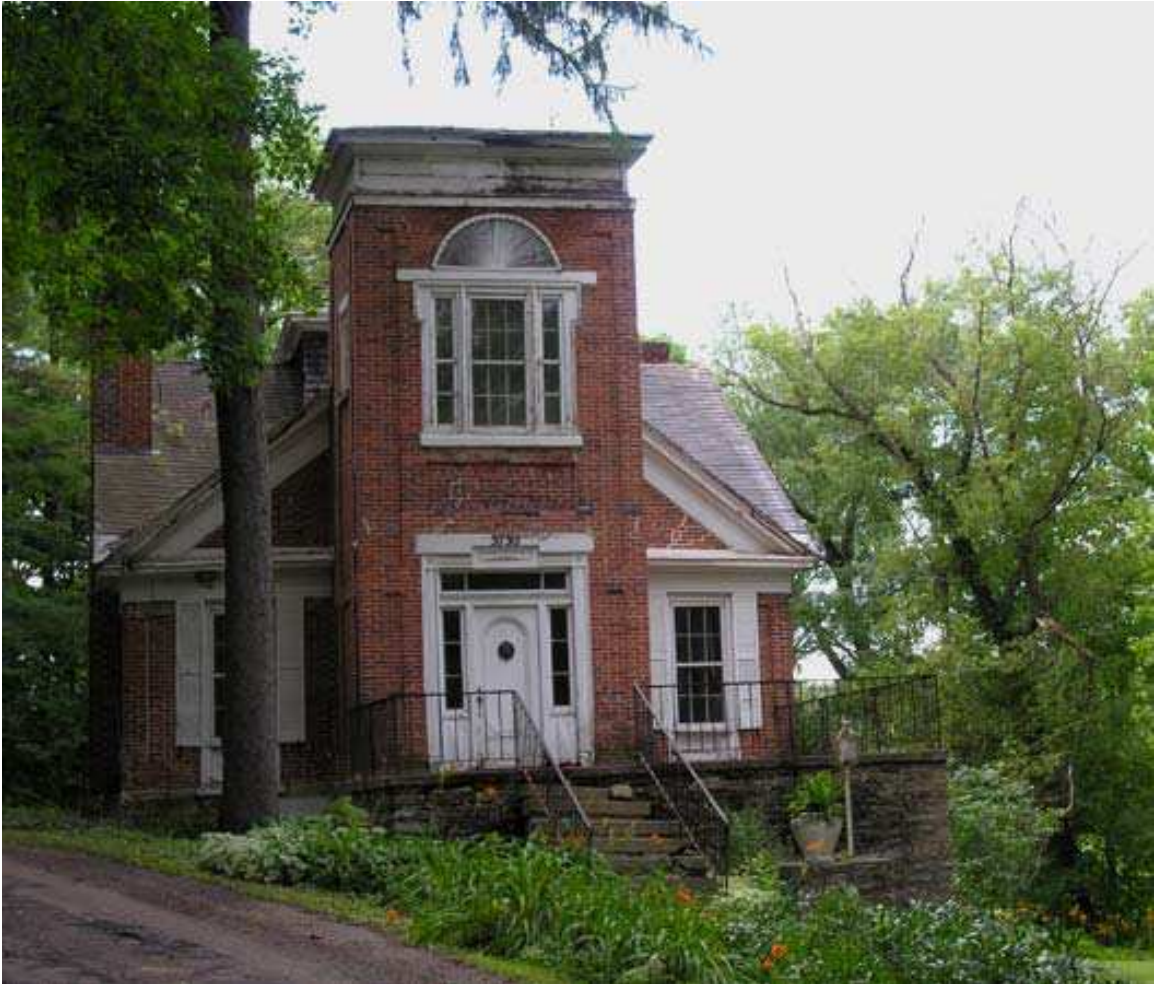
Figure 2. Front view of the Biermann house, 2010. Although the house is believed to have been built by John FitzJermole Harmon in the 1860s, Adolph Biermann likely added the Romanesque entry tower in the 1880s. The front terrace and garage were constructed in the 1930s, during a renovation of the house that prepared it to become the home of Alice Mayo's parents (see lower level floor plan for photo vantage point).
