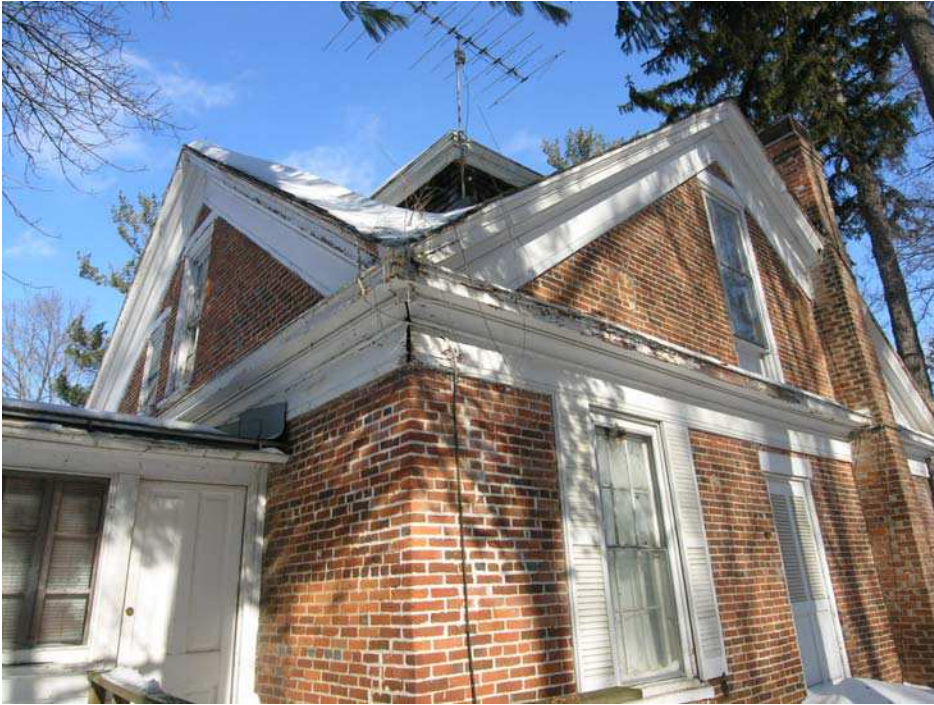
Southwest view. Note the house's cross gabled roof and the central tower, which has a skylight.
