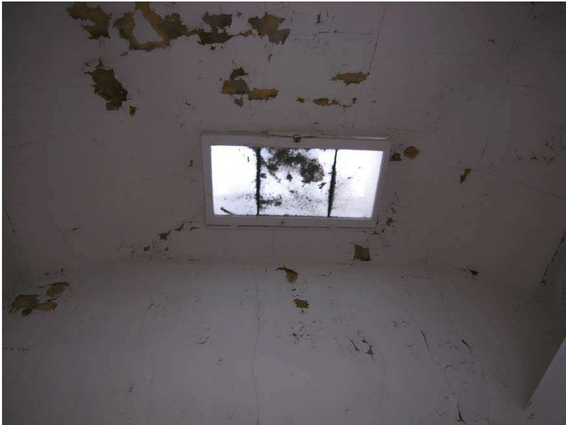
Skylight in the tower addition's upper level bedroom
