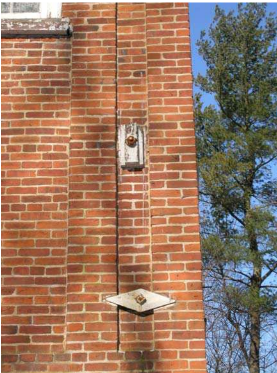
Stabilizing anchors in the entrance tower addition
