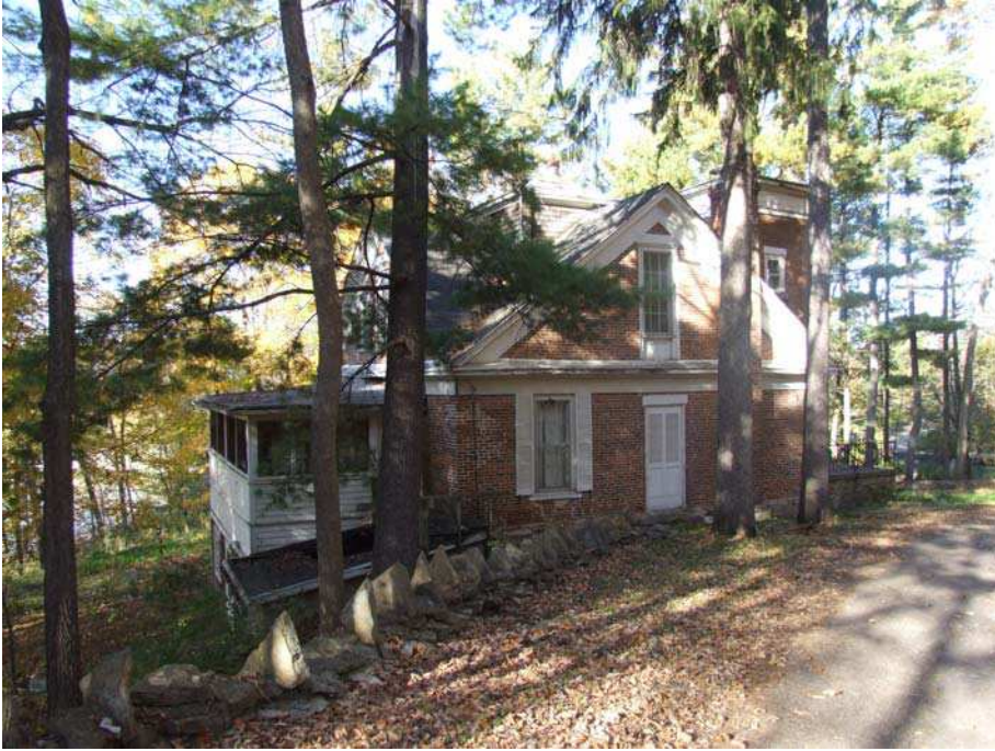
Figure 3. View of the house from the Mayowood driveway. Note the “dragon tooth” wall (see lower level floor plan for photo vantage point).
