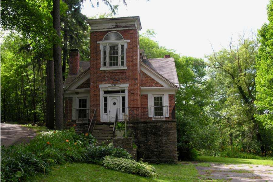
Figure 1. Front of the Biemann house, from lower level driveway (see lower level floor plan for photo vantage point).
