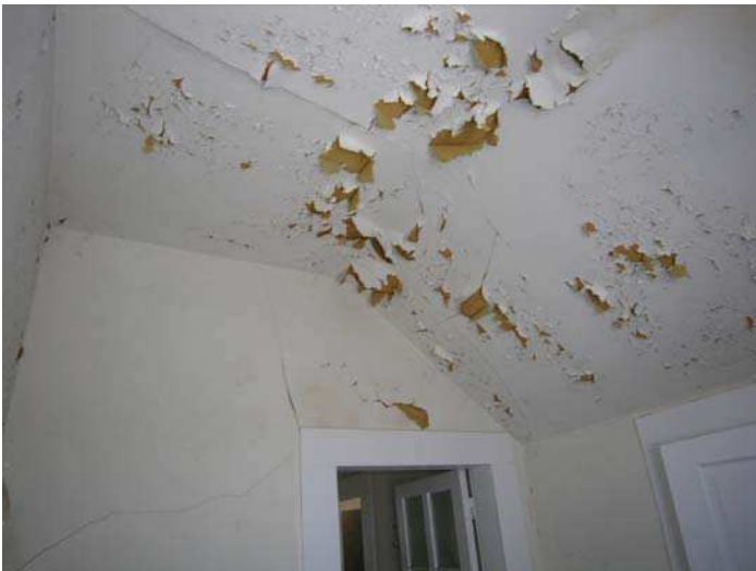
Upper level hallway ceiling
