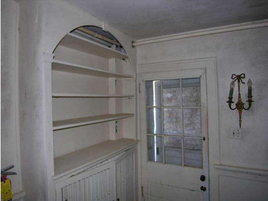
Lower level family room. Note the concealment of pipes and radiator within cabinetry.
