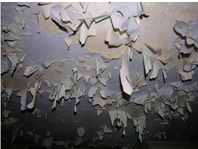
Lower level kitchen ceiling
