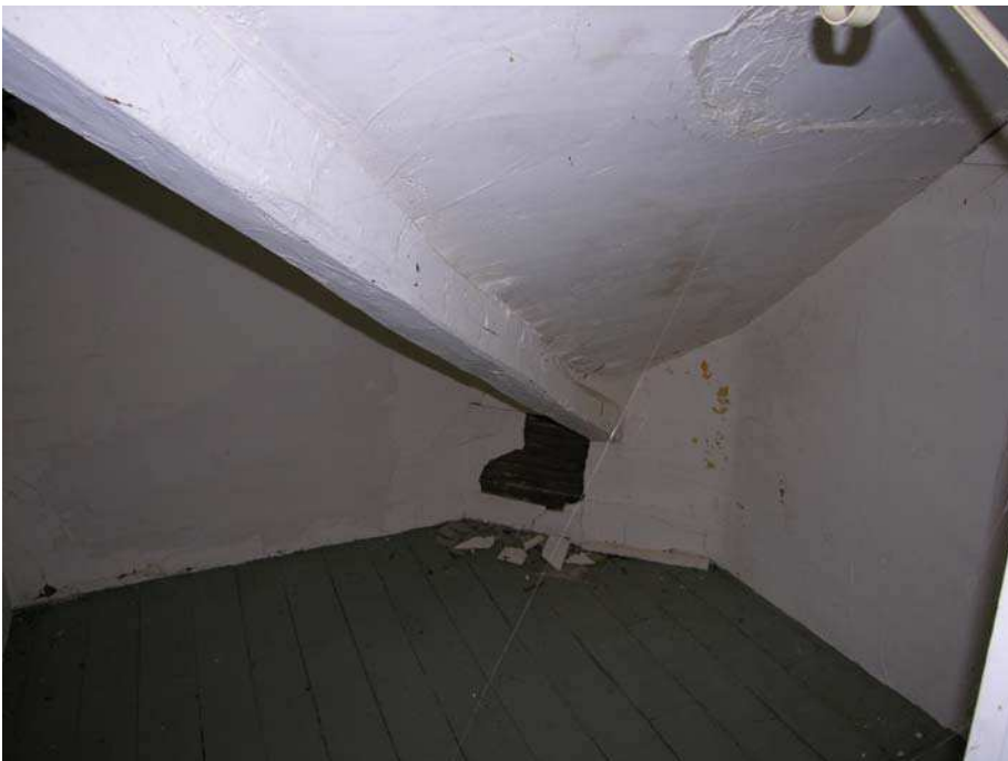
Upper level closet corner detail from stairs hallway
