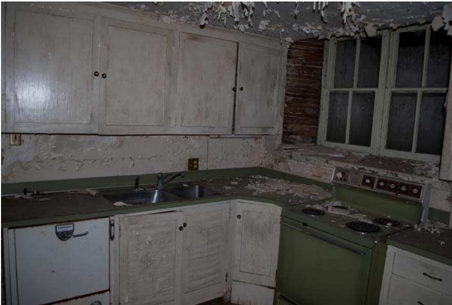
Figure 7. Lower level kitchen. This is believed to be the original kitchen location (see lower level floor plan for photo vantage point).
