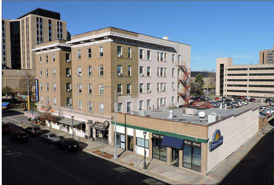
Figure 6. Southeast Elevation, Facing Northwest.
