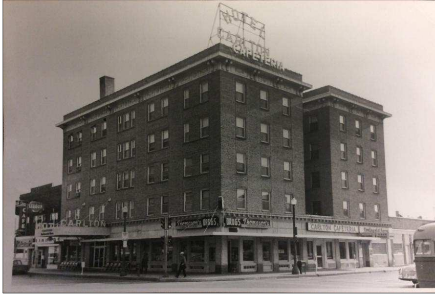
Figure 12. Hotel Carlton Southwest Elevation, Facing Northeast, 1939 (History Center of Olmsted County).
