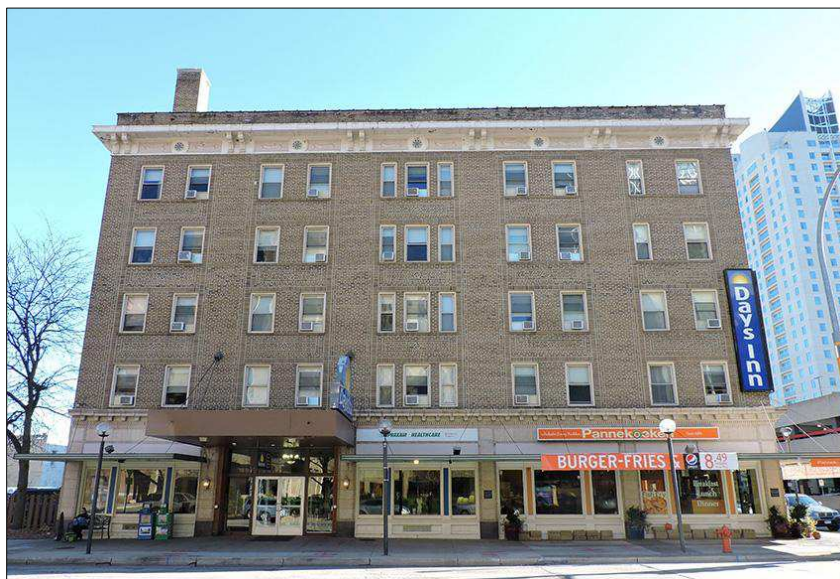
Figure 4. West Façade, Facing East.
