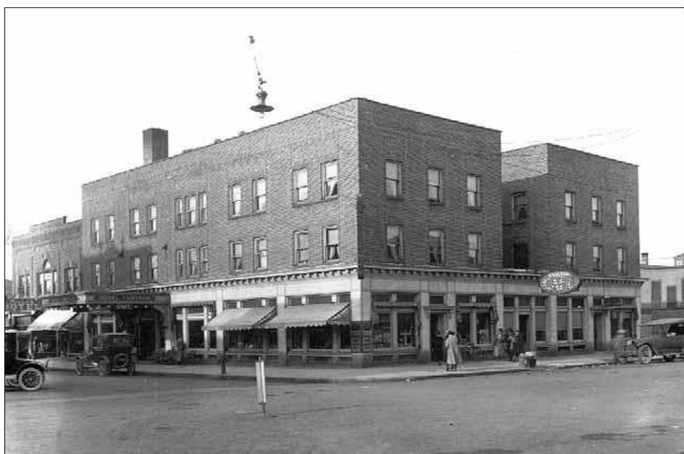
Figure 8. Southwest Elevation, Facing Northeast, c. 1925 (MNHS c. 1925).
