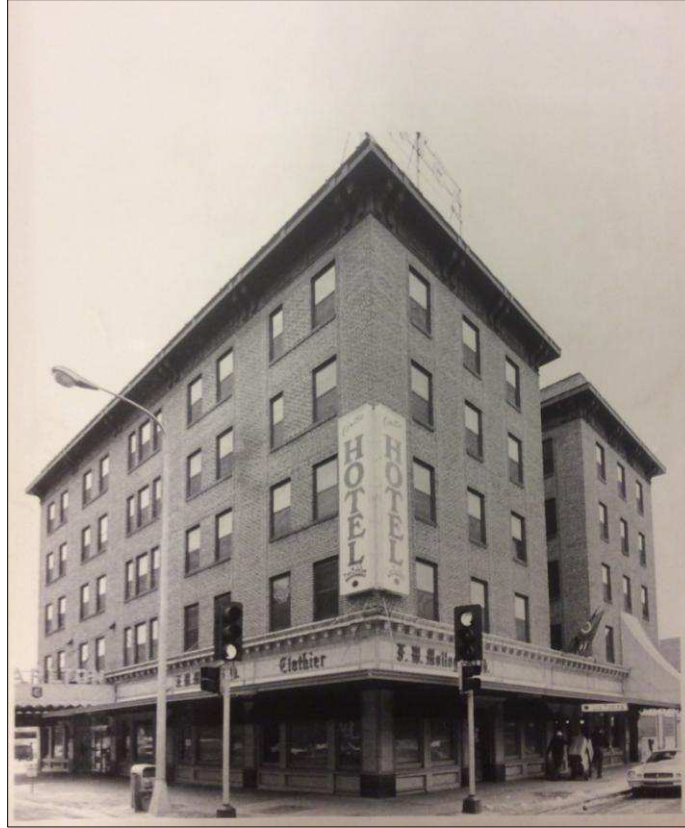
Figure 13. Hotel Carlton Southwest Elevation, Facing Northeast, 1983 (History Center of Olmsted County)
