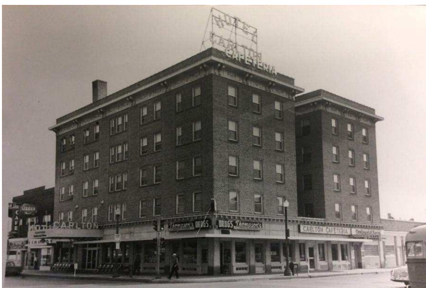
Facing NE, 1939 (History Center of Olmsted Co)
