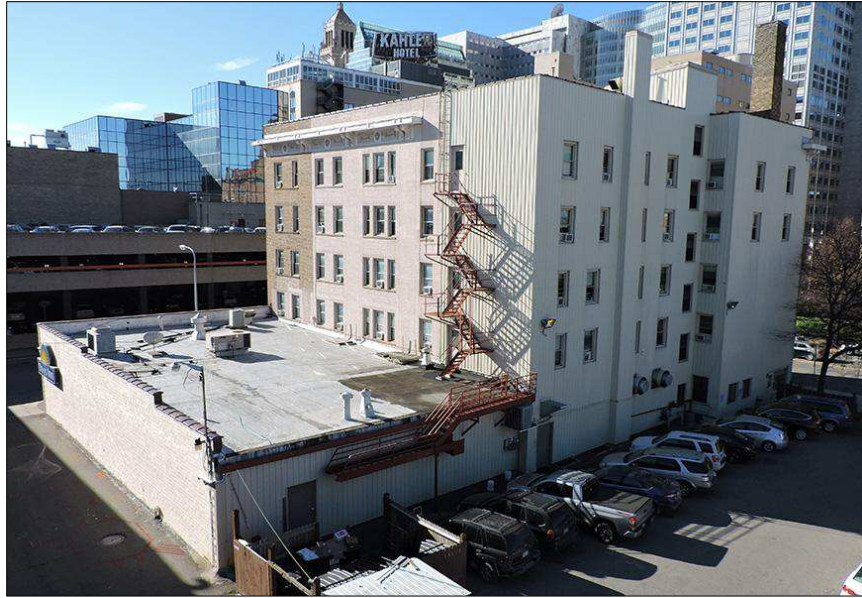
Figure 7. Northeast Elevation, Facing Southwest.
