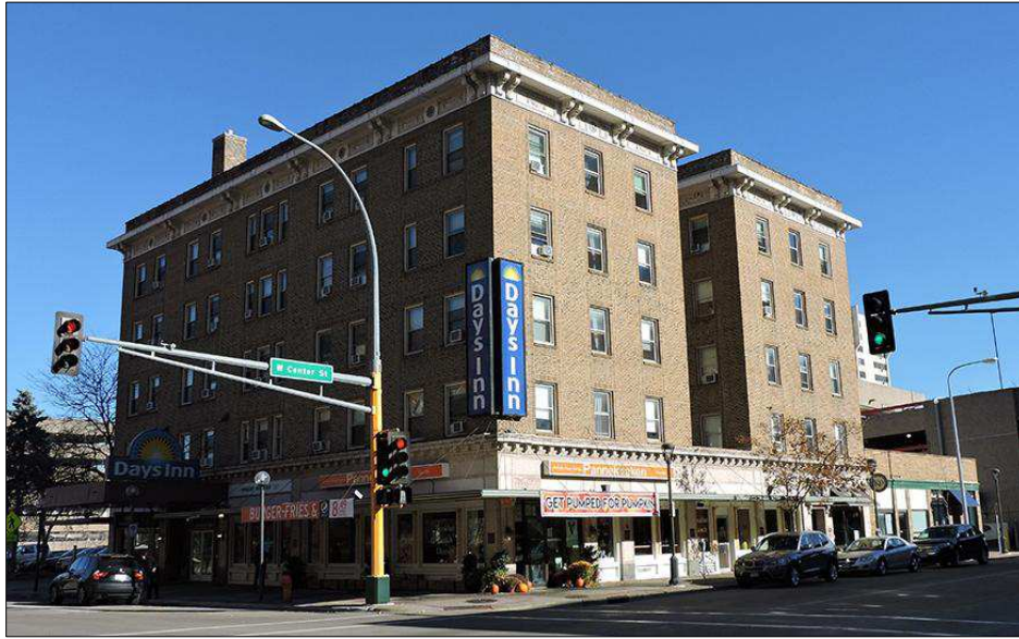
Figure 2. Hotel Carlton, Facing Northeast.
