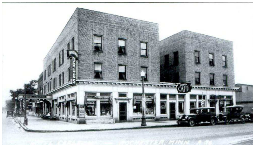
Figure 9. Southwest Elevation, Facing Northeast, 1925 (Calavano 2008:31).
